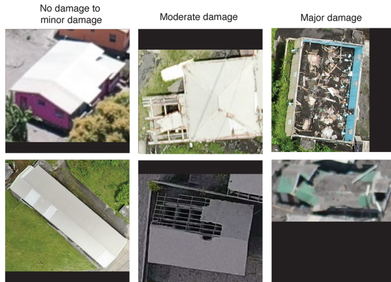
Figure 2. Example of the three damage states used in this work: No damage to minor damage, Moderate damage and, Major damage.
