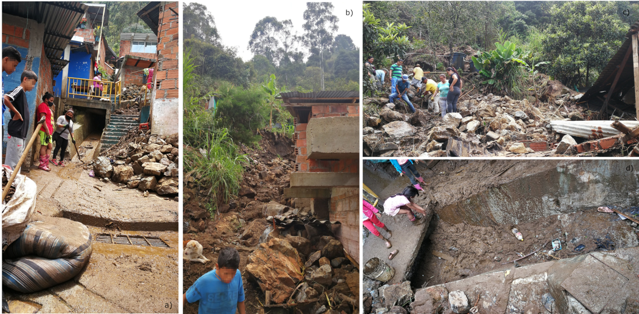
Figure 3. Pictures from the 2021 La Rafita Creek Flash flood event in El Pacífico. a) cleaning process of mud and debris by the community. b) household affected by the flood. c) Upper part of the neighborhood after the flash flood. d) mud in the lower portion of the neighborhood. Photos: Junta de Acción Comunal El Pacífico
