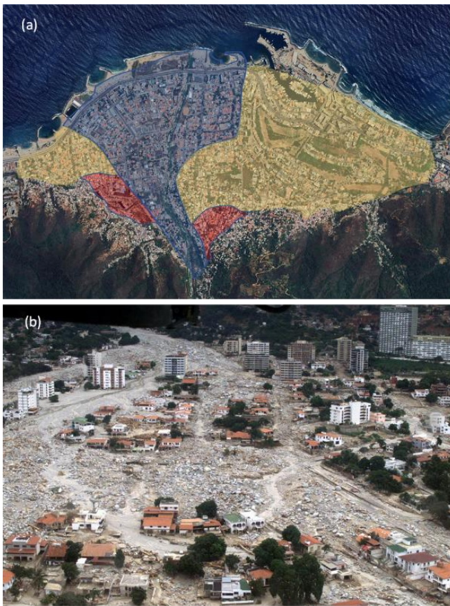
Figure 2: The 1999 Caraballeda flood. The debris flow impact 1.3 km 2 of the city. (a) flood deposits: blue, the 1999 flood; yellow, historic debris flow; and red, prehistoric deposits (Source: Wiczorek et al., 2001). (b) aftermath (source: Larsen and Wiczorek, 2006).
