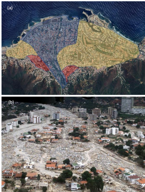
Figure 12: The 1999 Caraballeda flood. The debris flow impact 1.3 km 2 of the city. (a) flood deposits: blue, the 1999 flood; yellow, historic debris flow; and red, prehistoric deposits (Source: Wiczorek et al., 2001). (b) aftermath (source: Larsen and Wiczorek, 2006).
