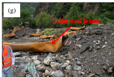
234 Figure 3. Photographs of the damaged residential buildings caused by debris flows during the field
