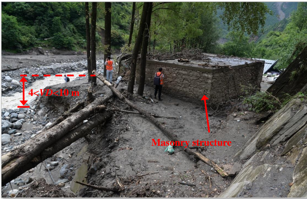
305 306 Figure 7. Example of the determination of the VD threshold, and VD in this figure indicates the height
