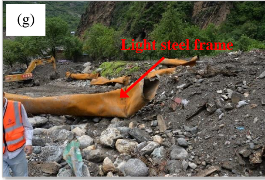
260 Figure 4. Photographs of the damaged residential buildings caused by debris flows during the field 261 investigations on the Qinghai-Tibetan Plateau
