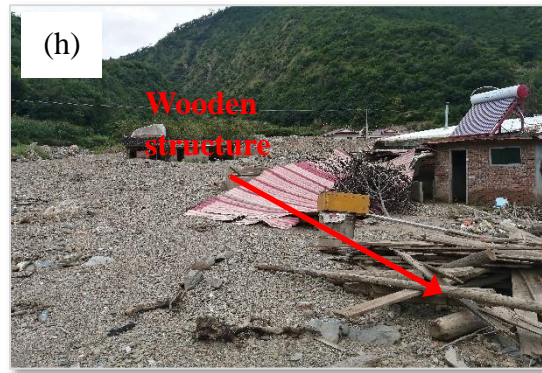
260 Figure 4. Photographs of the damaged residential buildings caused by debris flows during the field 261 investigations on the Qinghai-Tibetan Plateau
