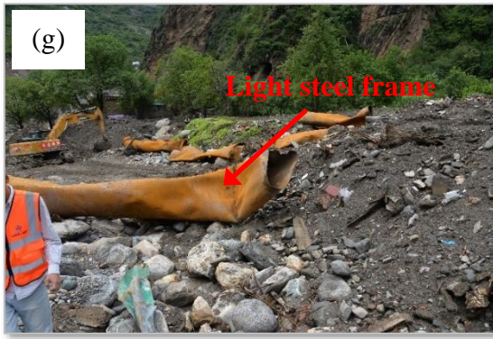
259 260 Figure 4. Photographs of the damaged residential buildings caused by debris flows during the field 261 investigations on the Qinghai-Tibetan Plateau
