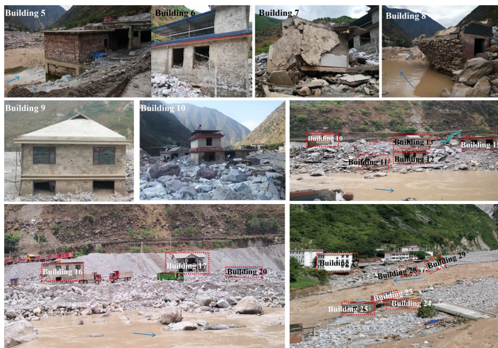
Figure 10 Buildings with the different degree of damages within three hazard zones.
