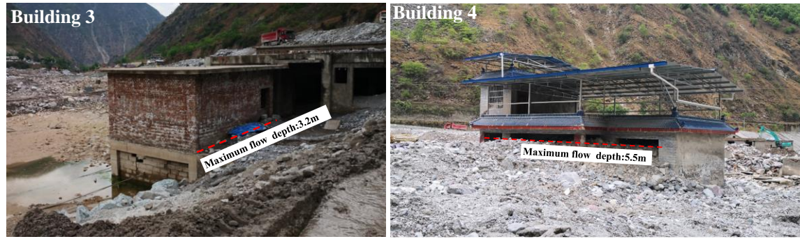
Figure 7 Simulated maximum flow depth of debris flow at the location of Building 3 and Building 4
