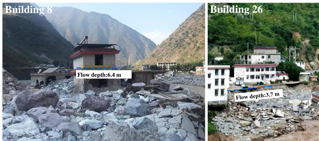
Figure 9 Simulated maximum flow depth of the dam-burst flood at the location of Buildings 8 and Building 26
