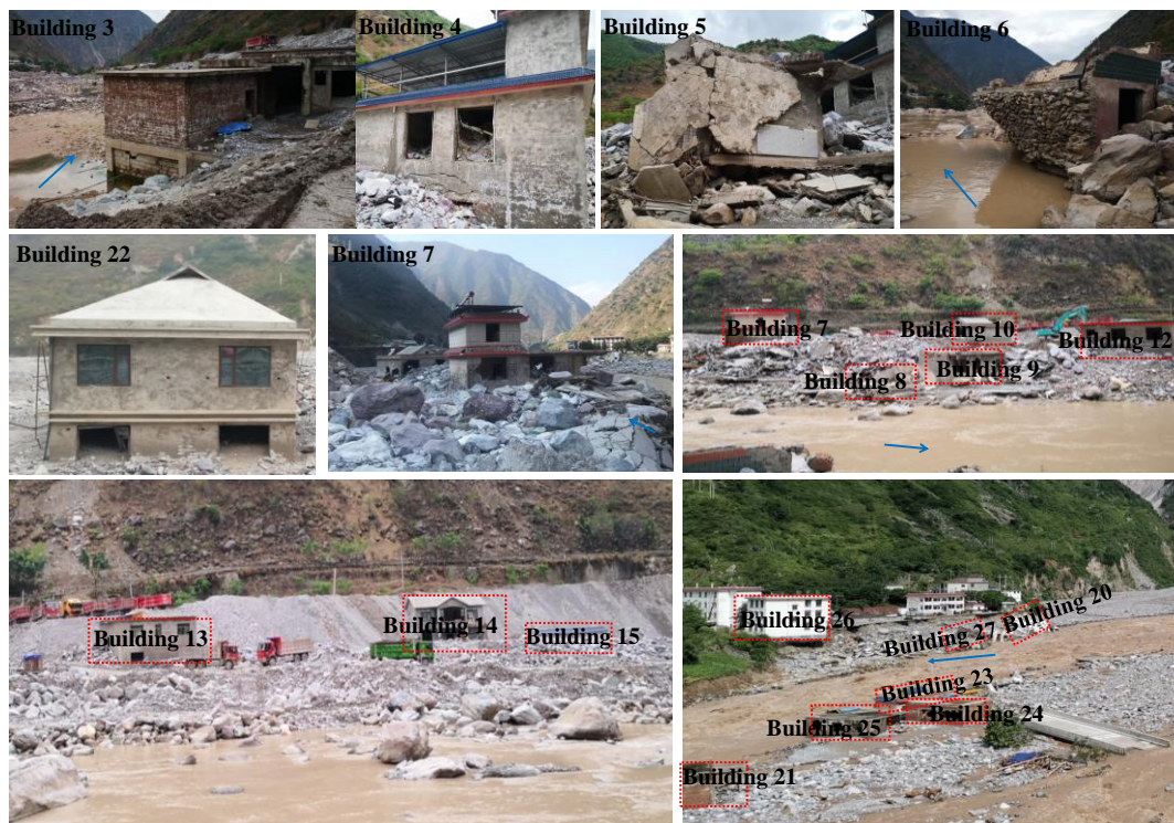
Figure 11 Buildings with different degrees of damage within three hazard zones.
