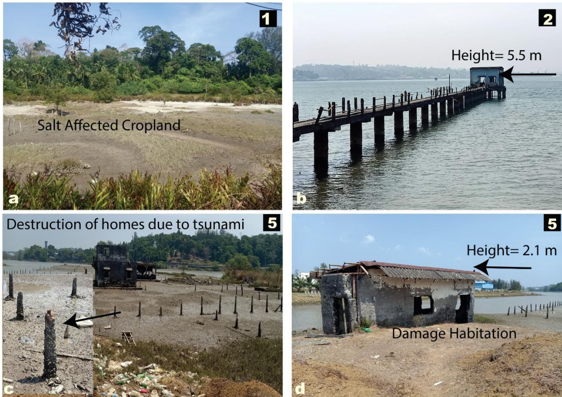
332 333 Figure 4: (a) Stagnation of Tsunami water in the agricultural field and Low-laying areas in Port Blair, (b) damaged 334 bridge in Bombooflat, (c, d) damaged house in the Sippighat area near Port Blair (Photo: 01/03/2023). The 335 number on the field photograph corresponds to respective locations, as in Fig. 3.
