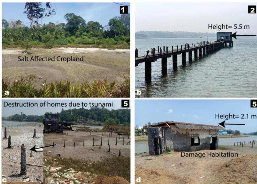
415 416 Figure 4: (a) Stagnation of Tsunami water in the agricultural field and Low-laying areas in Port Blair, (b) damaged 417 bridge in Bombooflat, (c, d) damaged house in the Sippighat area near Port Blair (Photo: 01/03/2023). The 418 number on the field photograph corresponds to respective locations as in Fig. 3.
