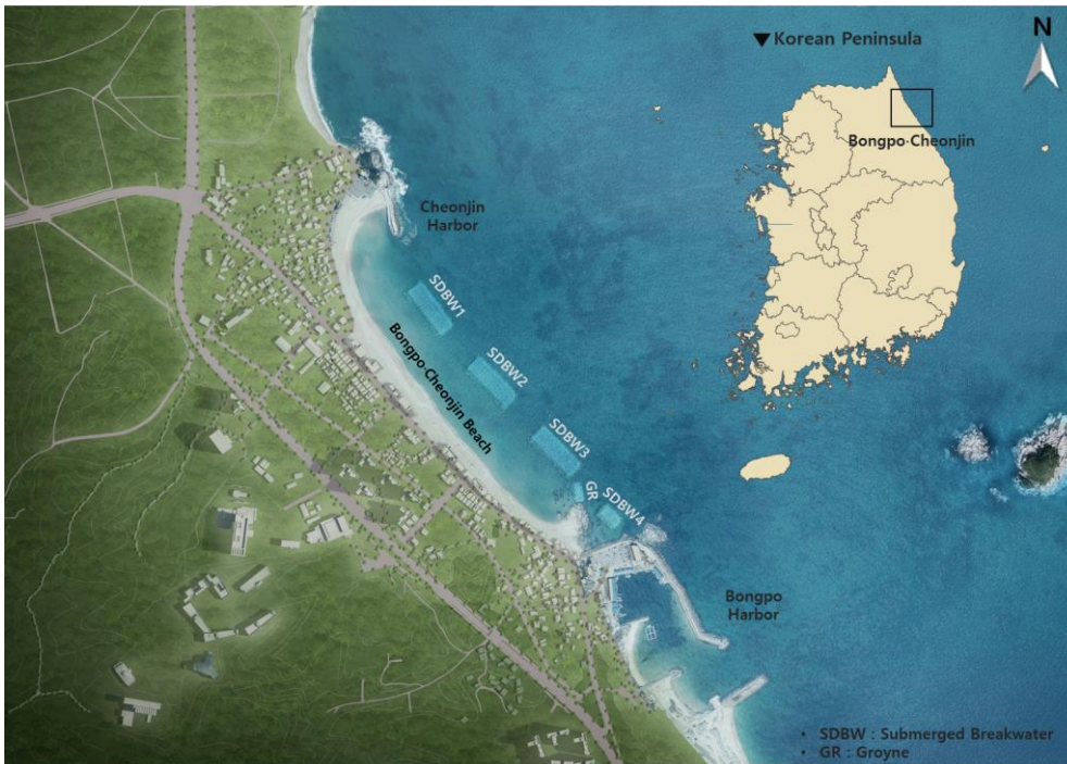
Figure 12: Location of Bongpo-Cheonjin Beach and coastal structures to mitigate beach erosion.
