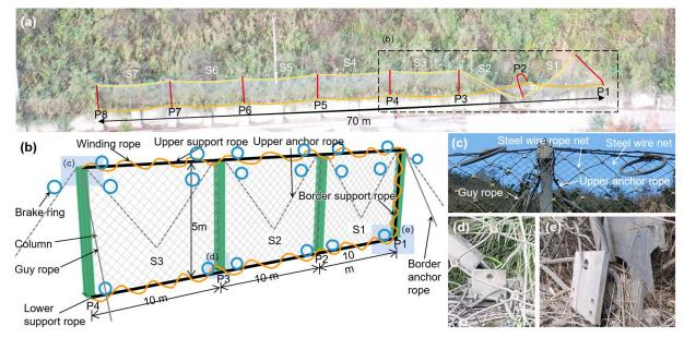
Figure 5: Structure composition of the flexible barrier. (a) Overall photo of the project; (b) Components connection relationship; (c) Column upper end; (d) Base and foot of column in the middle spans; (e) Base and foot of border column.
