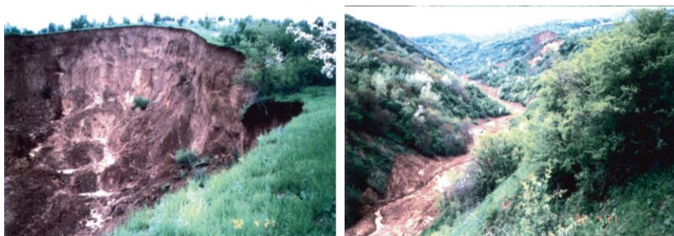
Fig. 12. Breakaway wall and mud flow along the Sharkilamasai (2002).
