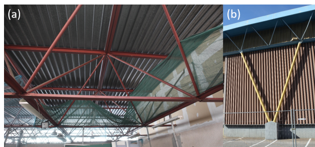
Figure 7. View of the supporting structure of the Irstea Cévennes building before its damage: (a) red-colored roof metal frame and (b) supporting tubular pylons (in yellow) along the facades.
