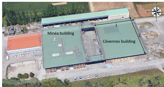
Figure 6. Overview of the Irstea Cévennes building before damage (Photo credit: ©Google Earth 2014, adapted by I. Ousset).
