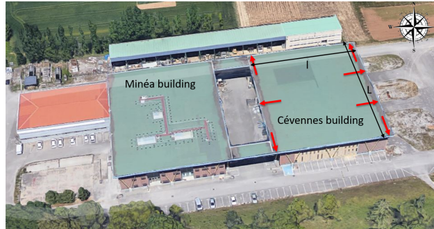
Figure 6. Overview of the Irstea Cévennes building before damage, with drainage points of rainwater indicated by red arrows (Photo credit: ©Google Earth 2014, adapted by I. Ousset).
