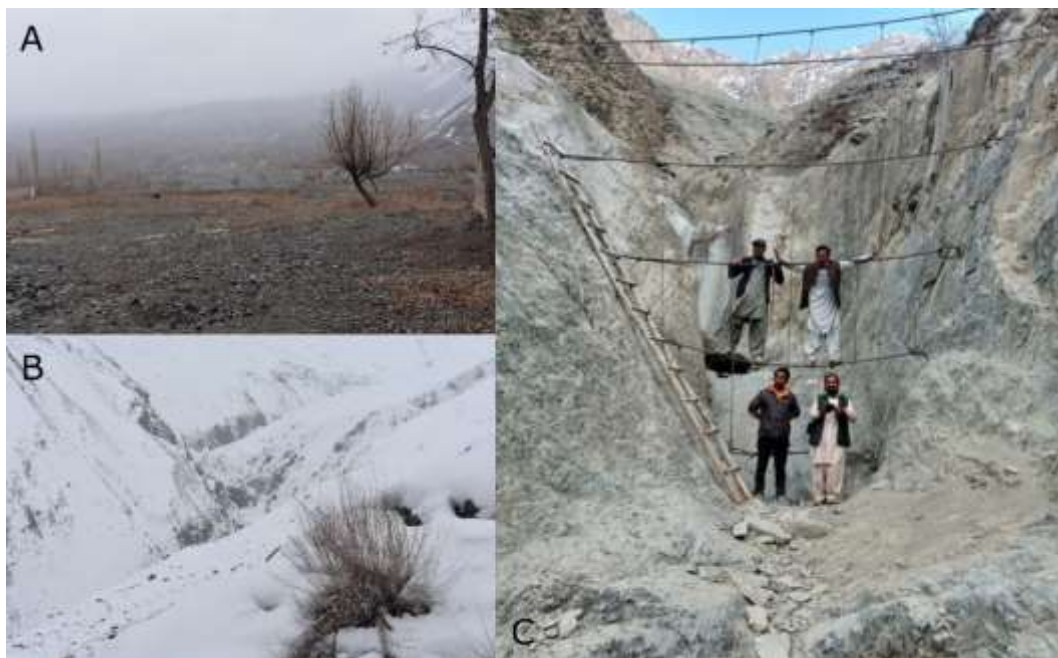
Figure 5: (A) Lower agricultural areas repeatedly at risk from avalanches but also in need of irrigation water. (B) The gully in March. (C) One of the multiple nets installed along the gully to capture avalanche snow.
