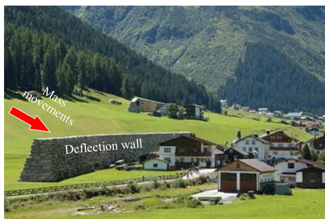
320 Figure 9. A deflection wall used to protect an entire building ensemble from the impact of medium magnitude events (Galtur Tschafein, Austria) (Holub et al., 2012).
