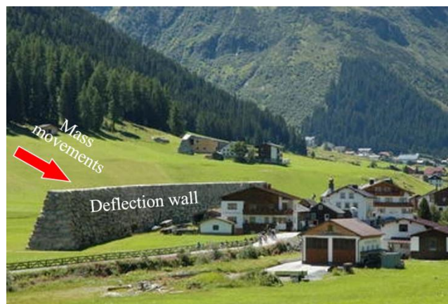
350 Figure 9. A deflection wall used to protect an entire building ensemble from the impact of medium magnitude events (Galtur Tschafein, Austria) (Holub et al., 2012).
