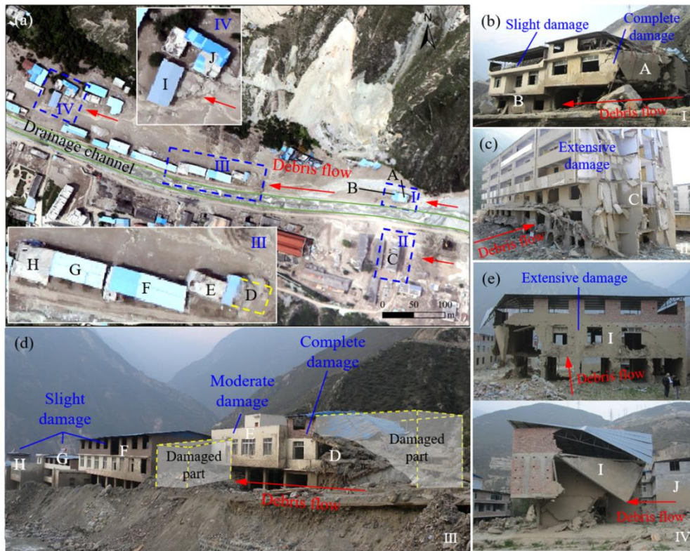
Figure 8. Distribution of damaged-buildings in Qipan gully debris flow event. Orthophoto map is from the Basic Geographic Information Center of Sichuan Province, China, 21 July 2013.
