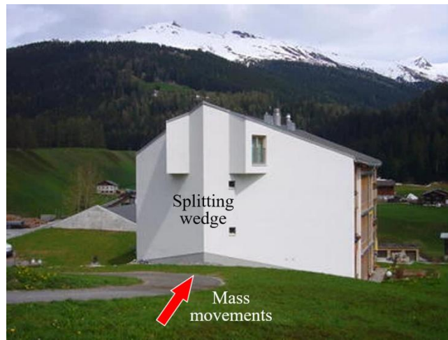
Figure 16. Splitting wedge directly connected to the exposed object (Davos Frauenkirch, Switzerland) (Holub et al., 2012).
