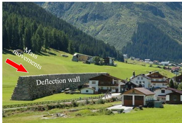
Figure 9. A deflection wall used to protect an entire building ensemble from the impact of medium magnitude events (Galtur Tschafein, Austria) (Holub et al., 2012).
