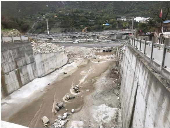
(c) discharge chute for debris flow
