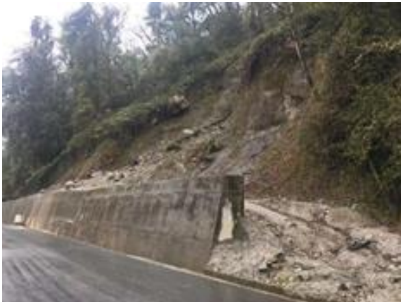
(a) gravity retaining wall
