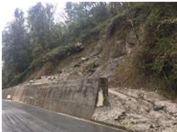
(a) gravity retaining wall
