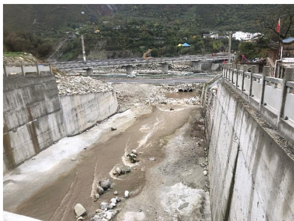
(c) discharge chute for debris flow
