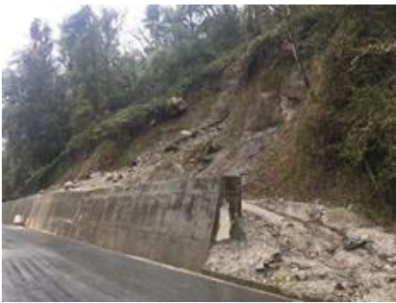
(a) gravity retaining wall
