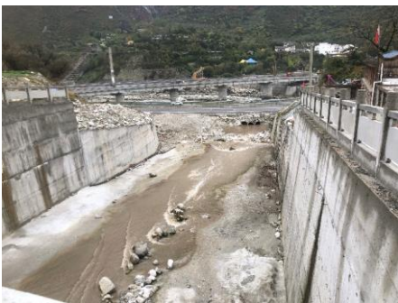
(c) discharge chute for debris flow
