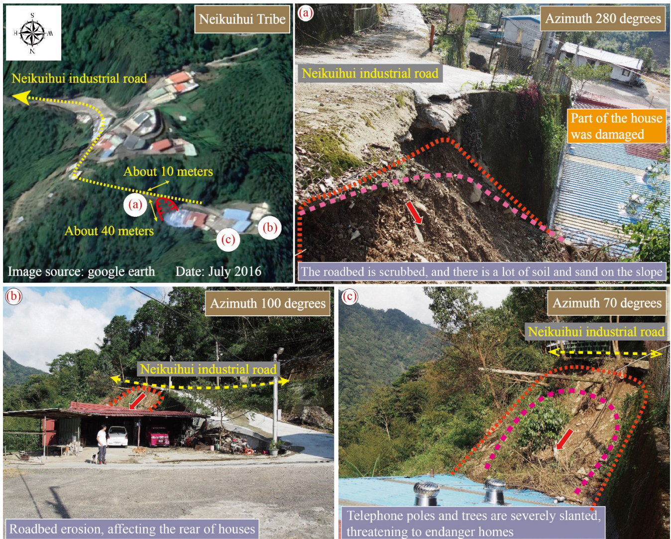
410 Figure 14 Historical disaster event at No.11 slope unit during Typhoon Meiji 2016 (Picture source: 2016 Water and Soil Conservation Bureau; Aerial: ESRI ArcGIS 10.4).
