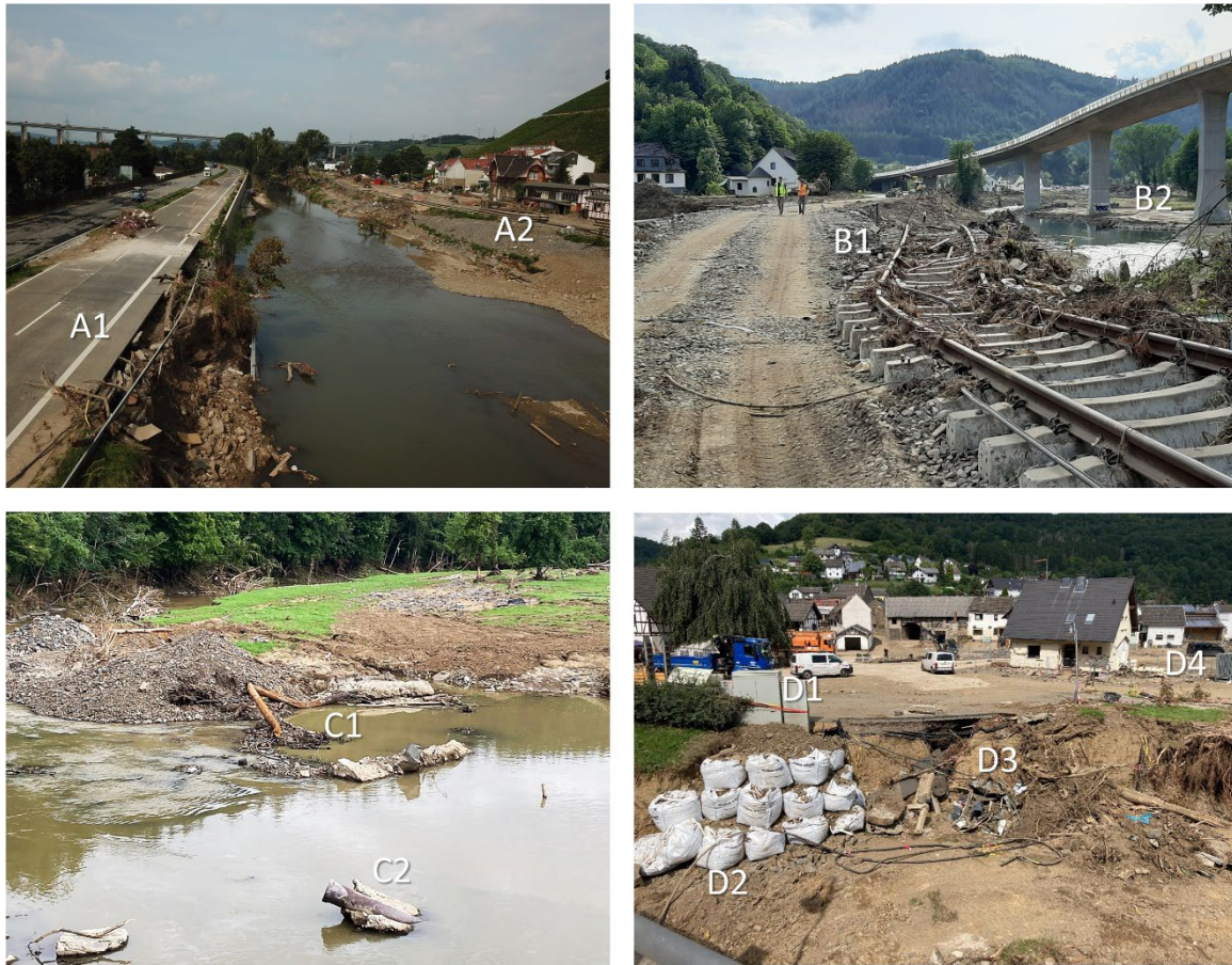
70 Figure 1. Damage in the Ahr Valley, Germany (images taken on 11 August 2021). Top-left: destruction of federal highway B266 (A1) and railway (A2) near Heimersheim. Top-right: further upstream in the Ahr valley (Altenburg), large stretches of the Ahrthalbahn railway have been destroyed (B1) and the few remaining road and rail bridges show signs of temporary repairs (B2). Bottom-left: river bed erosion uncovered and destroyed many cables supposed to lie more than 80 cm below surface level (C1) as well as sewers (C2). Bottom-right: inundated electricity distribution infrastructure (D1), road erosion and stabilisation (D2), uncovered cables (D3) and collapsed buildings in Schuld. Pictures by Margreet van Marle/Deltares/GEERassociation, distributed under Creative Commons Attribution 4.0 license.
