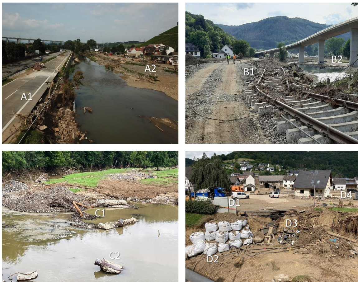
70 Figure 1. Damage in the Ahr Valley, Germany (images taken on 11 August 2021). Top-left: destruction of federal highway B266 (A1) and railway (A2) near Heimersheim. Top-right: further upstream in the Ahr valley (Altenburg), large stretches of the Ahrtalbahn railway have been destroyed (B1) and the few remaining road and rail bridges show signs of temporary repairs (B2). Bottom-left: river bed erosion uncovered and destroyed many cables supposed to lie more than 80 cm below surface level (C1) as well as sewers (C2). Bottom-right: inundated electricity distribution infrastructure (D1), road erosion and stabilisation (D2), uncovered cables (D3) and collapsed buildings in Schuld. Pictures by Margreet van Marle/Deltares/GEERassociation, distributed under Creative Commons Attribution 4.0 license.
