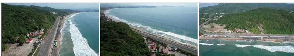
Figure 3: Aerial views of Boulevard Miguel de la Madrid.
