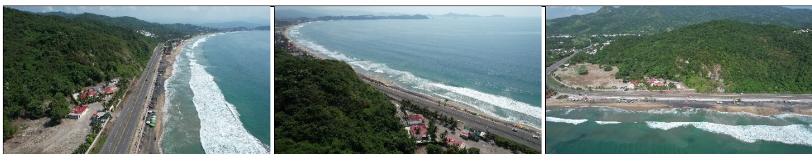
120 Figure 3: Aerial views of Boulevard Miguel de la Madrid.
