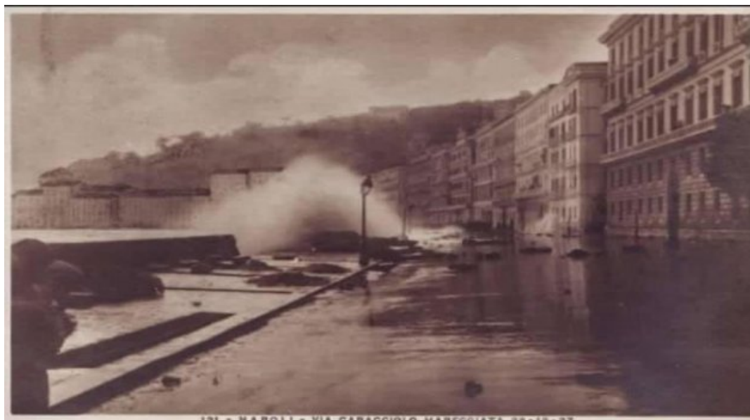
Figure 14. Historical photo of 1927-storm that impacted and destroyed via Caracciolo, Naples (from il Mattino newspaper).
