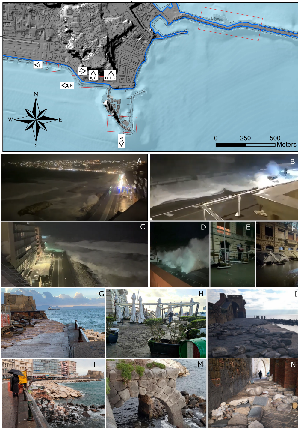
Figure 12. Photos of: A), B), C) and D) Storm surge in the coastal area with maximum setup values (Naples city center); E) and F) Damages on structures during the event; G) promenade destroyed with collapsed parapet; H) shattered shop windows; I) and N) Castel dell'Ovo after the event; L) and M) Bourbon pier after the event; H) Bourbon pier before the event. In the map, the onshore DTM from Lidar data was provided by Ministero dell'Ambiente; the offshore DTM derive from bathymetric data provided by Regione Campania.
