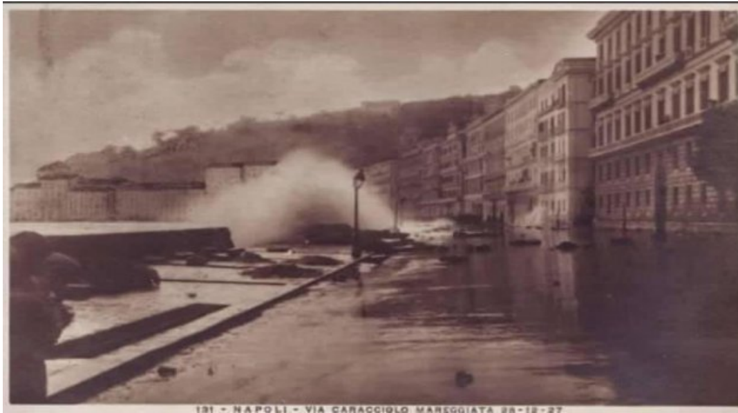
Figure 13. Historical photo of 1927-storm that impacted and destroyed via Caracciolo, Naples (from Il Mattino newspaper).
