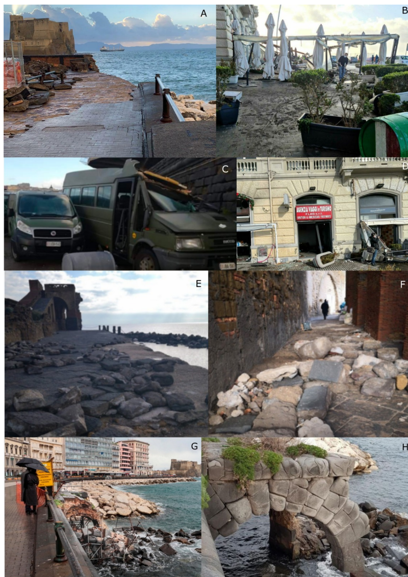
Figure 13. Photos of the main damages on structures after the event: A) promenade destroyed with collapsed parapet; B) damage on external structures of some restaurants; C) damage on military infrastructures; D) shattered shop windows; E) and F) Castel dell’Ovo after the event; G) Bourbon pier after the event; H) Bourbon pier before the event.
