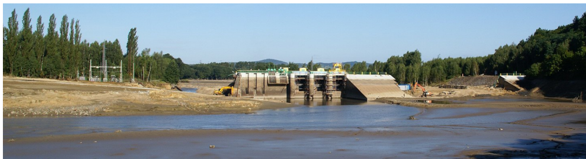
Figure 9. The final breach of the dam - an upstream view
