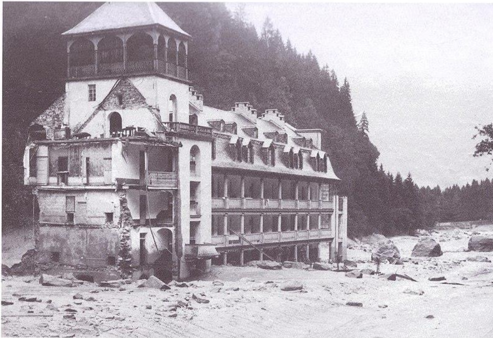
634 Figure A1. The wiped-out thermal bath of Saint-Gervais-les-Bains after the debris flow of the 12th of 635 July 1892 (Thermal bath establishment of Saint-Gervais, via www.thermes-saint-gervais.com ).
