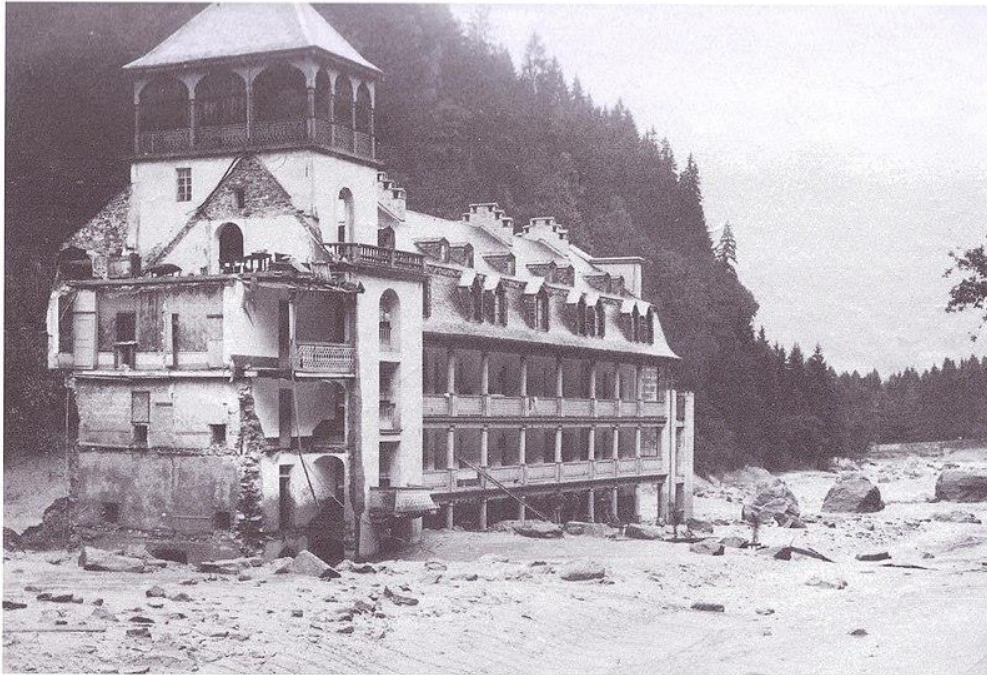
638 Figure A1. The wiped-out thermal bath of Saint-Gervais-les-Bains after the debris flow of the 12th of 639 July 1892 (Thermal bath establishment of Saint-Gervais, via www.thermes-saint-gervais.com ).
