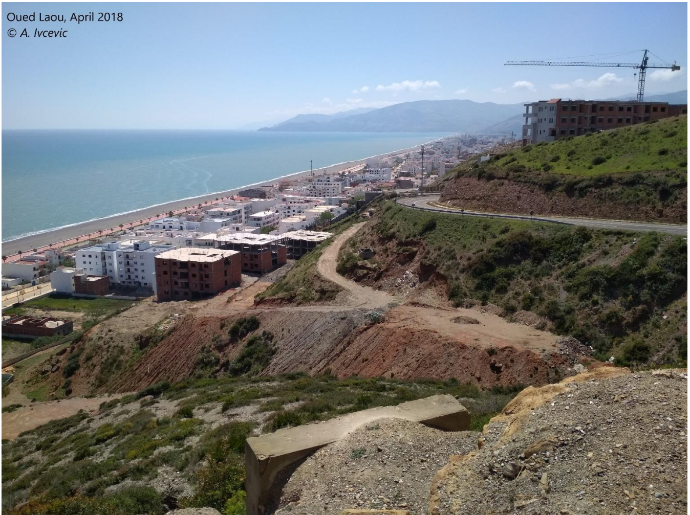
Figure 2: The region of North Morocco has a high increase of touristic infrastructure.
