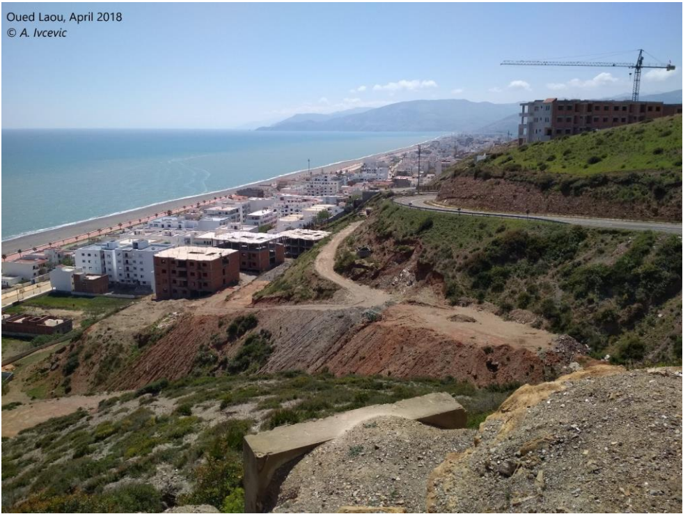
Figure 22: The region of North Morocco has a high increase of touristic infrastructure.
