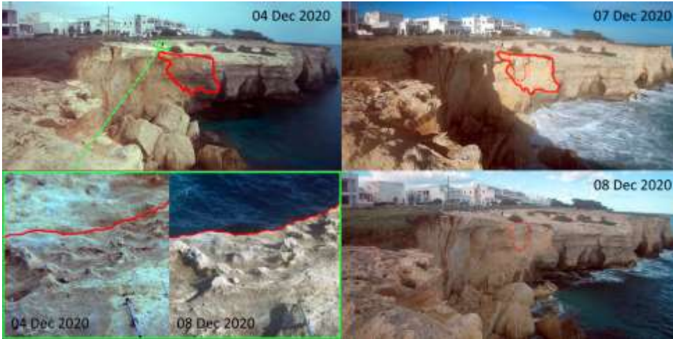
Figure 3: the second rockfall (marked with “B” on fig. 1) – Top left image shows the cliff as it was on 4 December 2020 and the top right image shows as it was on the morning of the 7 December 2020, after the main collapse (marked by the thick red line). Bottom right images shows the cliff as it was on the 8 December 2020, after a minor rockfall (marked by the thin red line). Those three images are taken from the secondary camera (see fig. 1 for the position). On the bottom left part, two smaller images that shows the collapse from another point of view (the main camera, that could also be seen in the top left image, highlighted in green – see fig. 1 for the position ) both before the rockfall (on the left) and after it (on the right). On those images, the newly installed automatic crackmeter is also visible.
