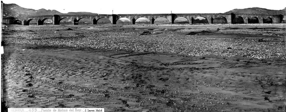
540 Fig.10 Bridge close to town D, shot by well-known French photographer Jean Laurent probably in 1866-1867. The only bridge in lower Llobregat at that time had a total length 334,36 metres, with 15 arches, the central 9 of which spanning 19,22 m each. It failed in 1971. Note the extremely wide alluvial area full of sand and gravel.
