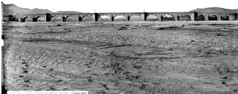
Fig.9 Bridge close to town D, shot by well-known French photographer Jean Laurent probably in 1866-1867. The only bridge in lower Llobregat at that time had a total length 334,36 metres, with 15 arches, the central 9 of which spanning 19,22 m each. It failed in 1971. Note the extremely wide alluvial area full of sand and gravel.
