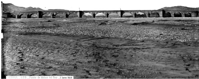
Fig.10 Bridge close to town D, shot by well-known French photographer Jean Laurent probably in 1866-1867. The only bridge in lower Llobregat at that time had a total length 334,36 metres, with 15 arches, the central 9 of which spanning 19,22 m each. It failed in 1971. Note the extremely wide alluvial area full of sand and gravel.
