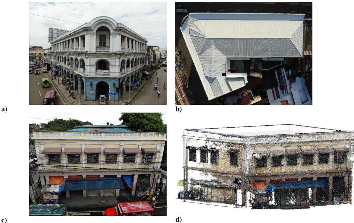
**Figure 6: Use of new technologies for the survey of the Iloilo City CH assets: Villanueva building front façade (a), and roof (b) by drone; Villanueva building 6 frontal façade (c) and point cloud (d) by drone and photogrammetry respectively.**
