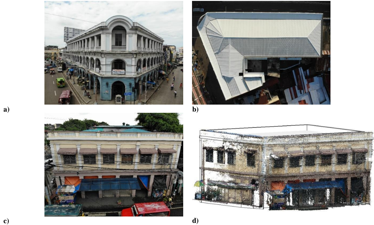
Figure 6: Use of new technologies for the survey of the Iloilo City CH assets: Villanueva building front façade (a), and roof (b) by drone; Villanueva building 6 frontal façade (c) and point cloud (d) by drone and photogrammetry respectively.
