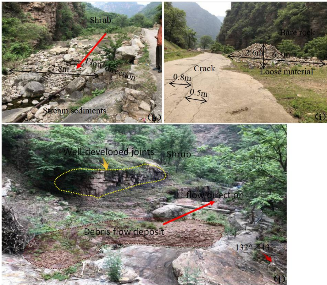
Fig.5 Lishu scenic spot. h stream sediments, i road cracks, g debris flow deposit.
