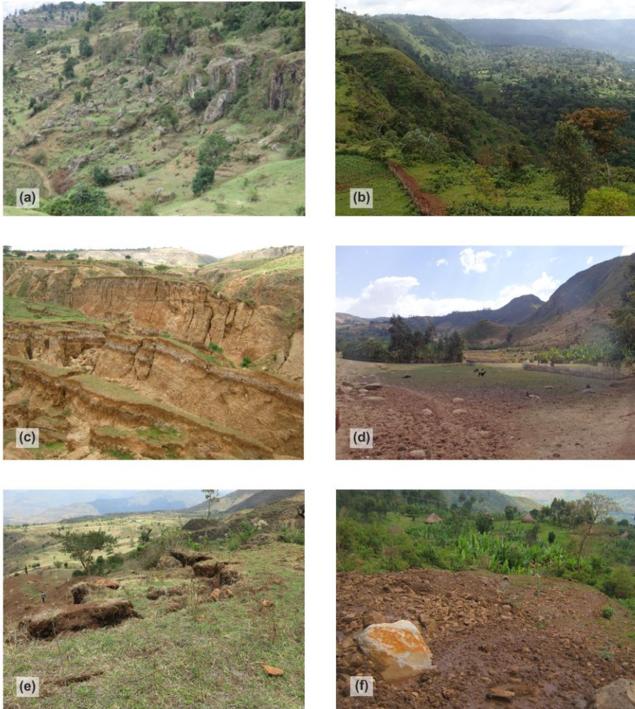
341 ▲ Fig. 7. Field photographs of various types of geohazards in MER – Hossana and Dilla areas. (a) Toppling and 342 subsequent rock fall of welded ignimbrites in the crown of a deep-seated landslide situated close to a fault scarp in 343 the western highland area (Dilla area; NW of Arba Minch town). (b) Large landslide in Dilla area (5 km SW of 344 Mejo town). (c) Tilted blocks of deep-seated landslide southwest to Awassa. (d) Undrained depression in the deep- 345 seated fossil landslide east of Dilla Town. (e) Tension cracks in the crown of a shallow landslide reactivated by road 346 construction, west of Arba Minch. (f) Recent debris flow accumulation below road construction in the landslide area 347 west of Mejo. 348
