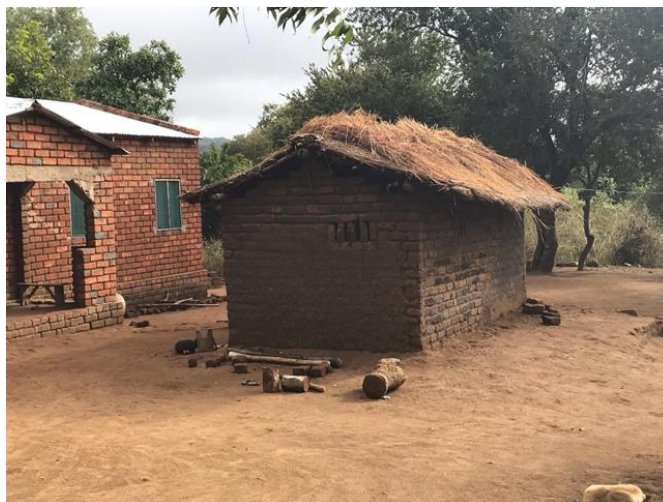
175 Figure 3: Image from one of the sample buildings taken in the case study area (Teule et al., 2019) A clear contrast between building material is visible between the two structures: hatched roofs and unburnt bricks versus iron sheeted roofs and burnt bricks.
