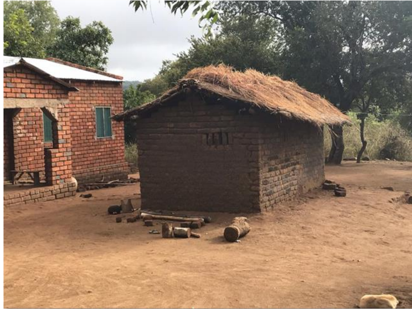
Figure 2: Image from one of the sample buildings taken in the case study area taken by T. Teule (23-06-2019). A clear contrast between building material is visible between the two buildings: thatched roofs and unburnt bricks walls (middle building) versus iron sheeted roofs and burnt bricks walls (left building).
