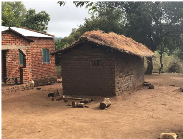
Figure 3: Image 2: image from one of the sample buildings taken in the case study area (taken by T. Teule et al., (23-06-2019)). A clear contrast between building material is visible between the two structures: thatched roofs and unburnt bricks walls (middle building) versus iron sheeted roofs and burnt bricks.
